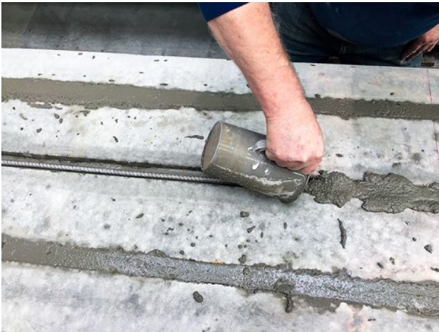
Versterking in sleuf
